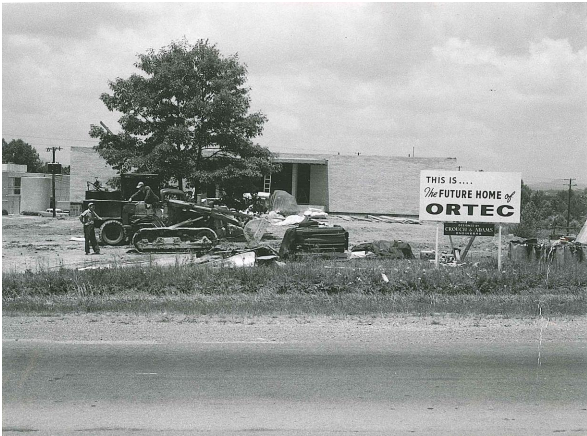
ORTEC begins construction on its first real home in 1963, a new building at 100 Midland Road and fronting on South Illinois Avenue
